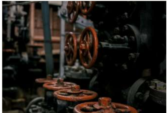
APPLICATION Row of red valve handwheels on industrial pipework — illustrative environment, not an installation of this product Illustrative scene
