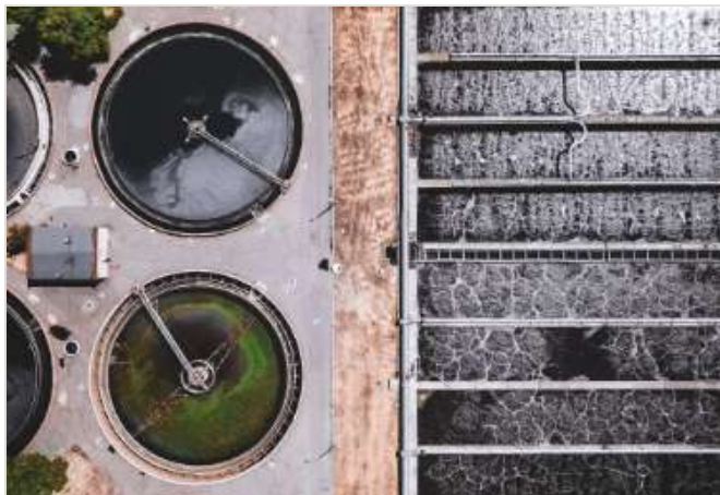
APPLICATION Aerial view of clarifiers and filter beds at a water treatment works — illustrative environment, not an installation of this product Illustrative scene
